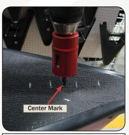
3. Find the center of the four marks and mark that center point. Use the 1-3/8" hole saw to drill out the center hole.
